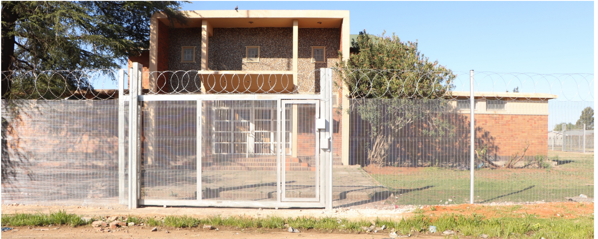
Jewel being restored: Florianville Civic Hall
